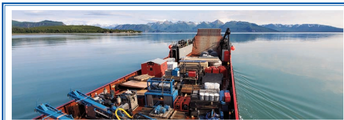
Drill equipment barged across Cook Inlet for the Johnson Tract Project (JT). The 2021 JT exploration program was completed with 19 of 44 drill holes released to date. Drill holes are from infill and expansion drilling at the JT Deposit.
